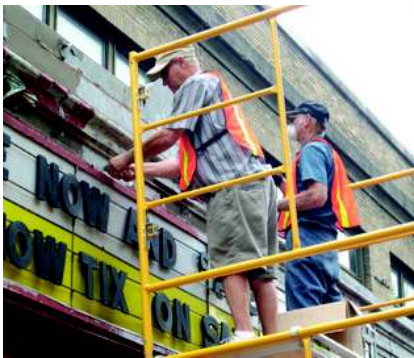
Craig Cristopher and Les Freeman of Cayuga Sign scraping old paint from the marquee.
